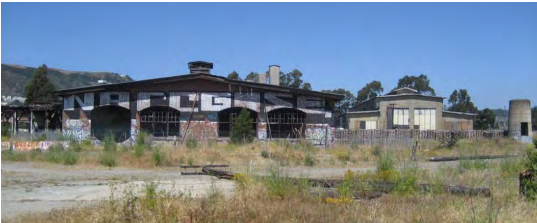
Figure 4.A-2e: Extant Historic Railroad Buildings on the Project Site. Looking northwest (facing away from the Caltrain tracks), the Roundhouse is on the left and the Lazzari Fuel Company building is on the right.
